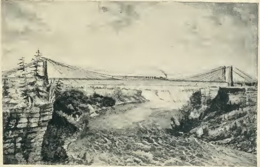
THE GRAND TRUNK RAILWAY SUSPENSION BRIDGE.
